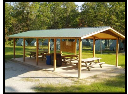
New campsite shelter
